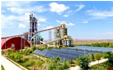
Wuzhong Saima New Type Building Materials Co., Ltd.'s "Photovoltaic + Smart Factory" project further enhanced the green and low-carbon transformation of the industrial park, adding new momentum to sustainable development.
