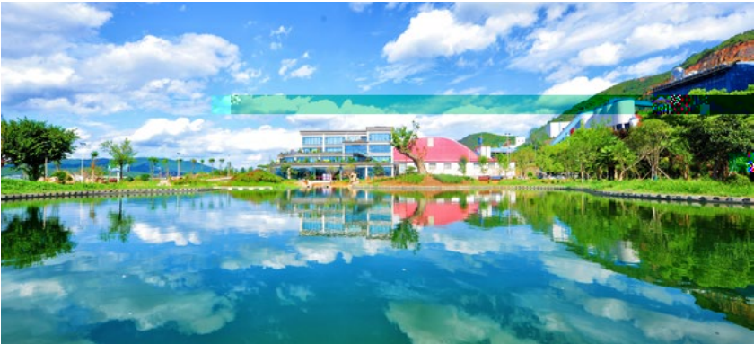
▲ The green factory of Xichuan Zhonglian Cements Co., Ltd.
